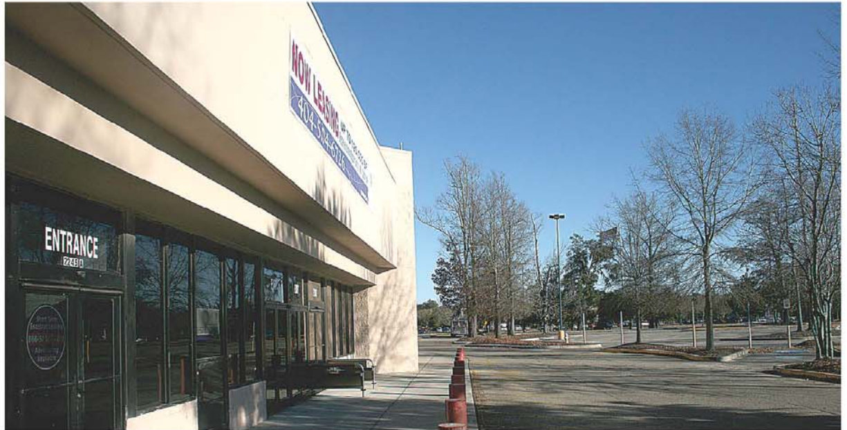
The old Wal-Mart building on Glen McConnell Parkway has been abandoned for years. But the West Ashley Senior Center could soon occupy the big empty space.
